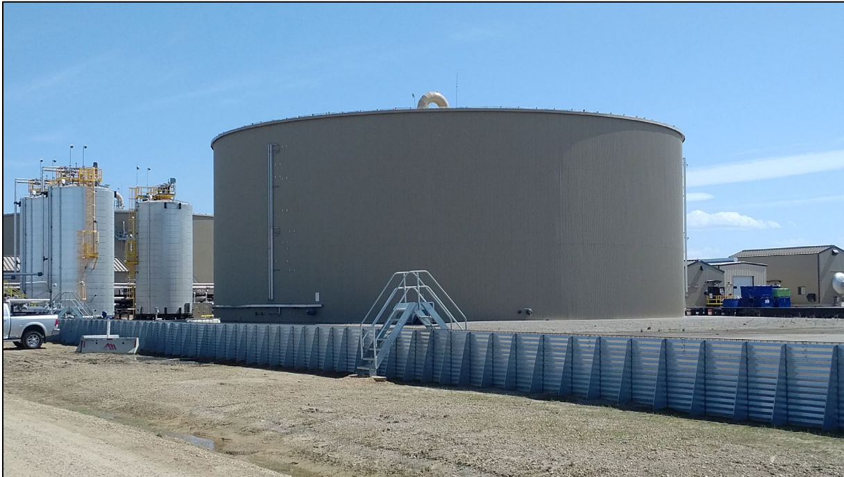
Figure 9. Industry water hub where hydraulic fracturing water is recycled and reused. Photo taken during the Panel's site visit.
