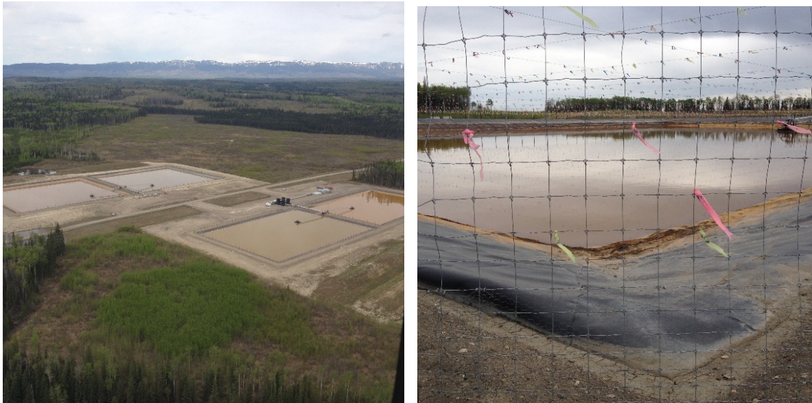
Figure 13. Containment pond for produced water. Aerial view (left) and close-up view (right) showing overhead and perimeter protection. Photos taken during the Panel's site visit.
